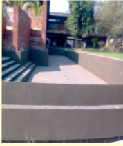
Swimming Pool Water Proofing System
