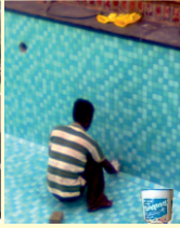
Glass Mosaic With Epoxy Grouting
