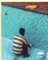
Glass Mosaic With Epoxy Grouting
